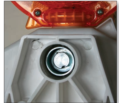
Recessed bolt hole to reduce theft of lights
