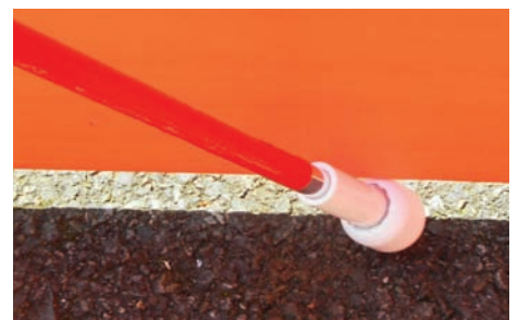
The bottom panel is 1.5" from the ground & acts as a detectable edge for pedestrians using canes.
