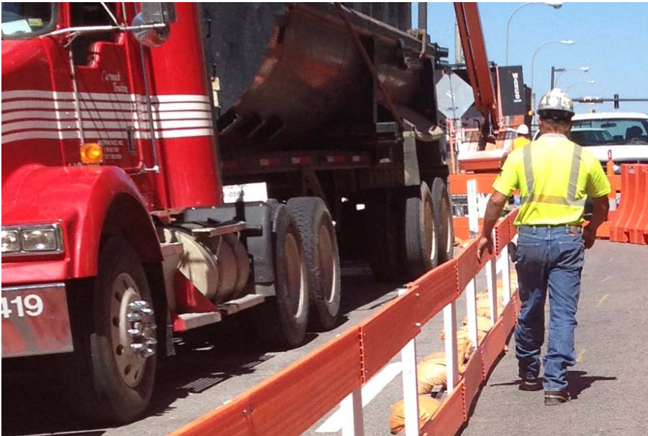
The top panel of the barricade acts as a smooth continuous guide for the hand.
