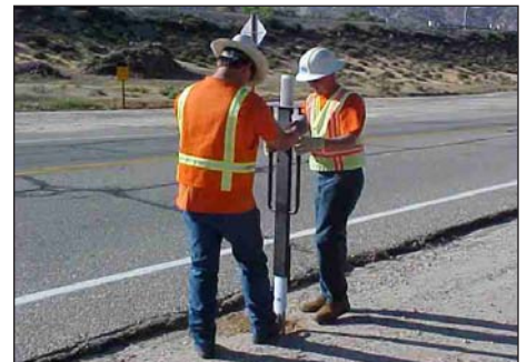
Both post styles are easily installed using an FG 103 Post Driver.
